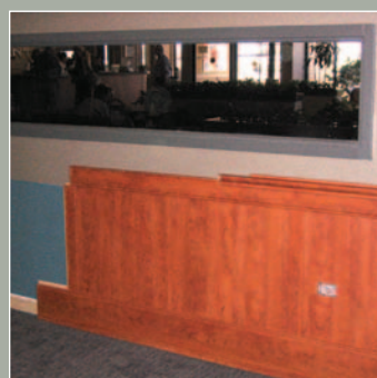
Apply top rail and rail cap
