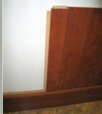
Level your base, slide stiles into grooves
