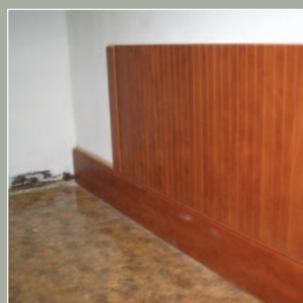
Slide panels in from the top
